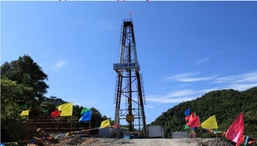
Deep drilling for uranium exploration project
