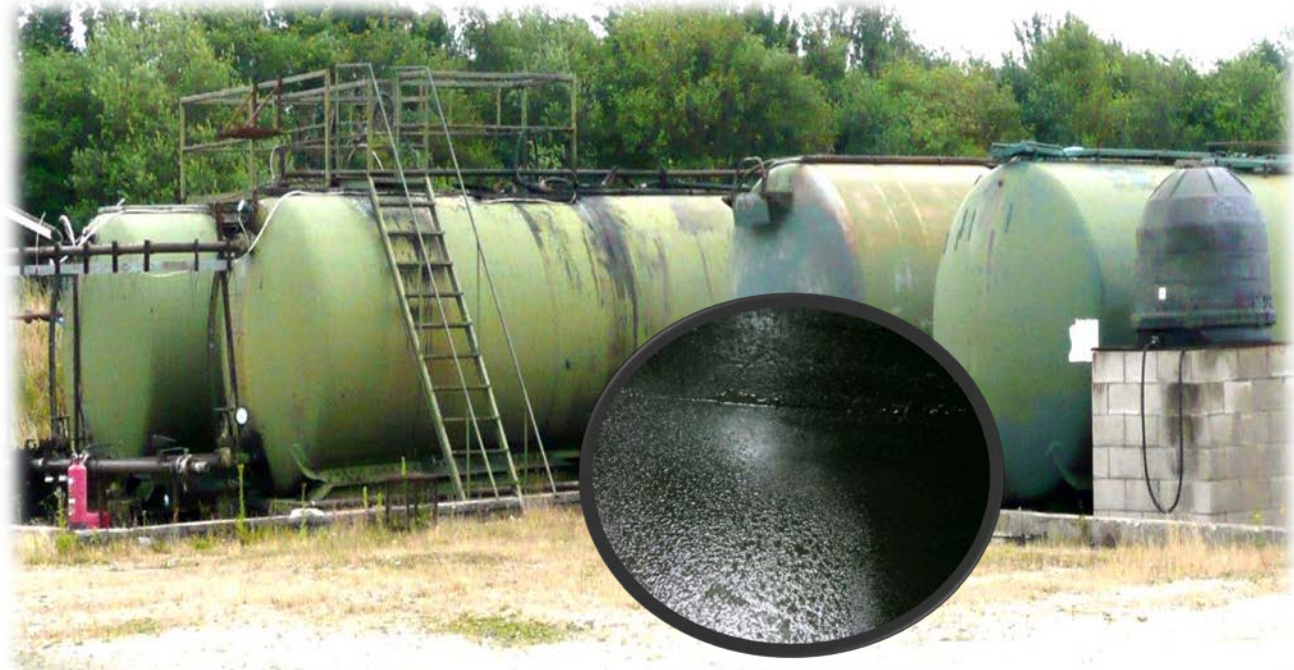
Removal of Heavy Sludges from Crude Oil Storage Tanks
