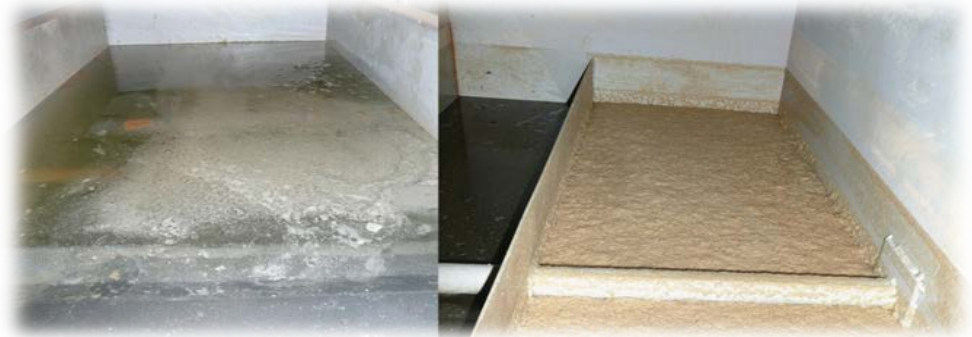
Gas Bubble and Floc Production in Flotation/Sedimentation Tanks
